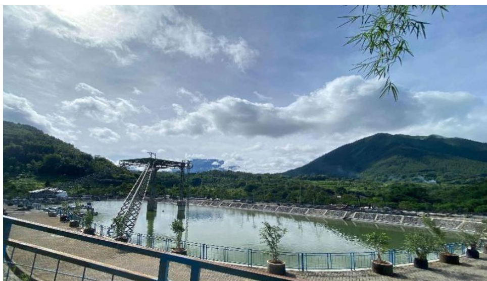
Figure 6.23 Implementation of Water Reservoirs
