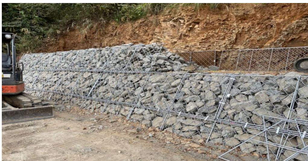
Figure 6.11 Gabion Check Dam
